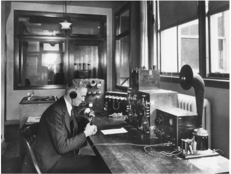
8MK / WWJ control room before Western Electric broadcast equipment was installed.
