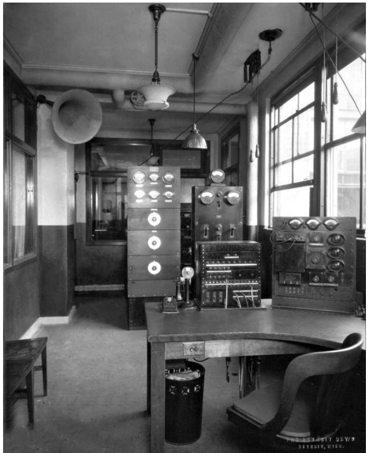
A somewhat later view of the WWJ control room showing more specialized transmitting equipment.
